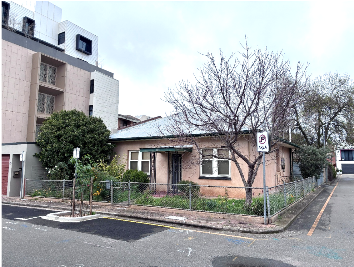
Figure 3.1 – Subject site from Wilson Street
